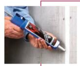
Flexible Firestop Protection for Fire Rated Joints.
