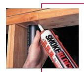
SmokeBlock® Caulk is a non-combustible caulking product that meets the requirements of ASTM E 136 for use in non-rated applications for fireblocking and draftstopping.
