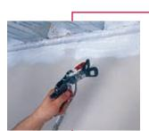
The Professional's Choice for Spray-Applied Firestop Protection of Joints and Penetrations.
